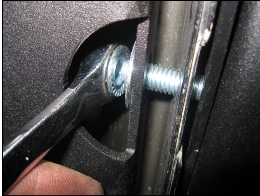
Figure 3. Using a closed-end wrench to hold each nut for tightening.
