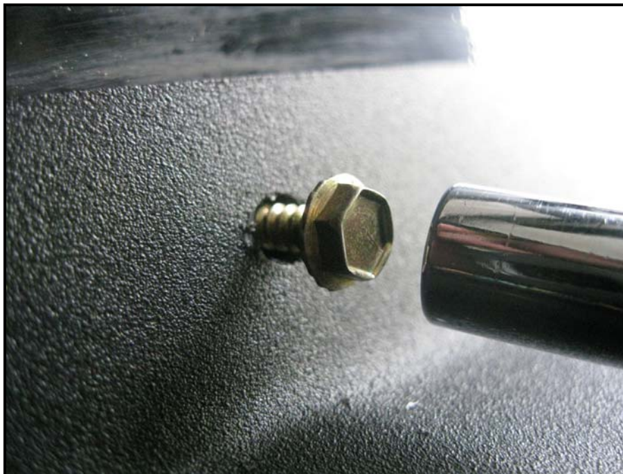
Figure 2. Use a 1/4" socket driver to install the Grip-Tight screws.
