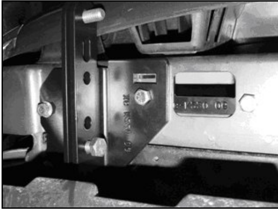
Photo 2. Passenger-side view (rear of vehicle toward bottom of image), showing location of inside mounting bracket and the backing plate visible through hole in crossmember.
